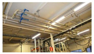
Panametrics has successfully provided accurate and reliable flow measurements on HVAC applications using either Transport PT900 or AT600 with C-RS for pipes above 2" and CF-LP (and upcoming CF-JR) for smaller lines as the illustrations demonstrate.
