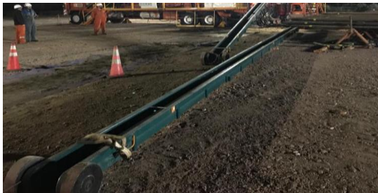
Two beams holding pre-assembled ESP unit at the wellsite.
