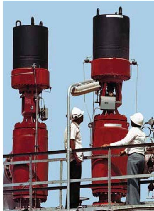
72000 Series Severe Service Control Valve
