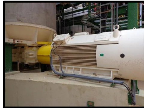
Figure 4 – HGF450 motor image. Source: Eldorado Brasil Celulose
