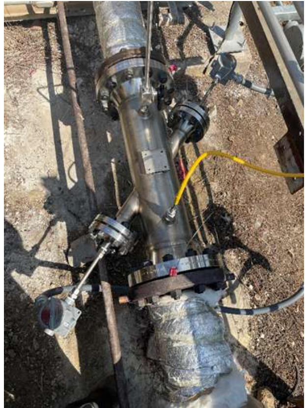
Panametrics ultrasonic steam flowmeter
