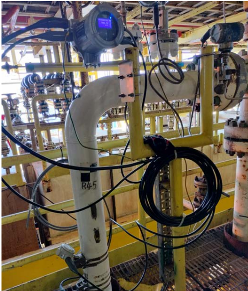
Fig. 2: PanaFlow LC and XMTXP R10 installation
