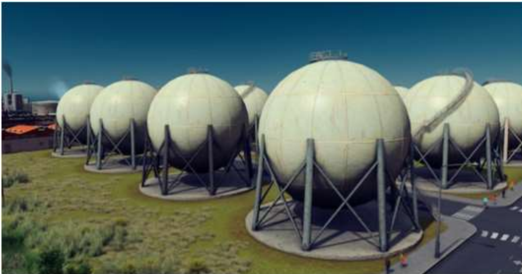
Figure 2: Spherical above ground storage tank farm – example of components that can be inspected on inside with remote control Bike platform
