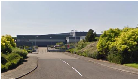
Data Center, Stone, UK
