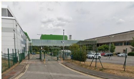
Data Center, Gloucester, UK
