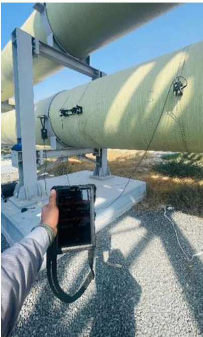
PT900 with CRR 591 0.5 Mhz transducers on DN1200 GRP pipe (48")
