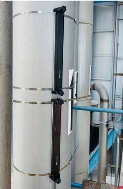
AT6-AT-10 transducers (1Mhz) on DN600 (24") HDPE pipe
