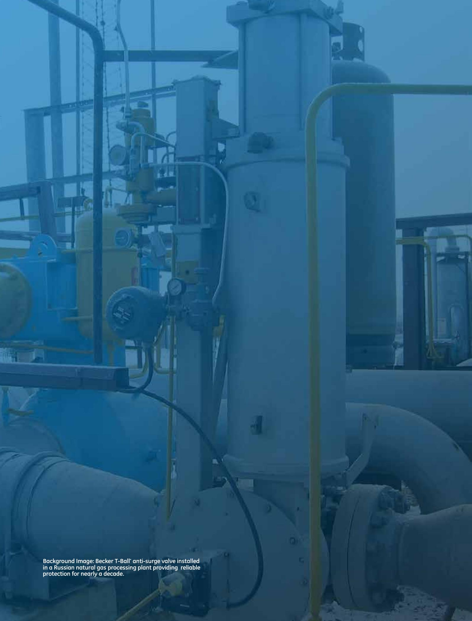
Background Image: Becker T-Ball® anti-surge valve installed in a Russian natural gas processing plant providing reliable protection for nearly a decade.
