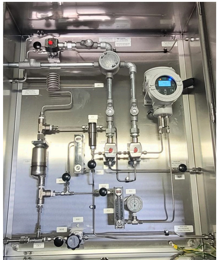
Figure 9: Sample system for tank blanketing
