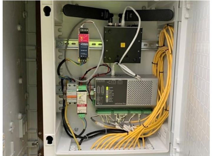
Fig 23: VB Online Pro monitoring system installation
