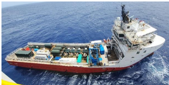
Baker Hughes assembled a temporary stimulation plant on this supply vessel for this challenging deepwater offshore job.
