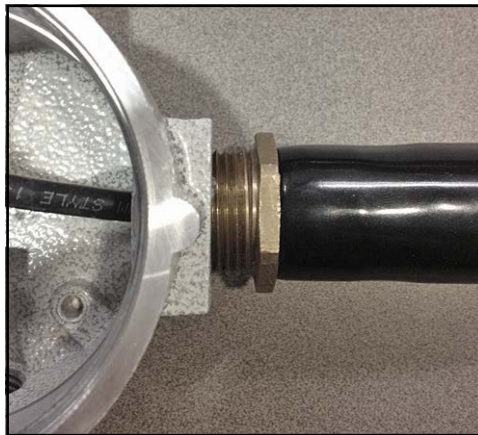
Figure 9: Torquing the Cable Gland
