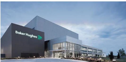
The Artificial Lift Research and Technology Center in Claremore, Oklahoma, USA features six vertical test wells, and offers enhanced, state-of-the-art system performance testing.
