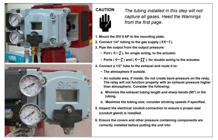
Figure 67 - Step 4 Connect Gas Supply and Exhaust
