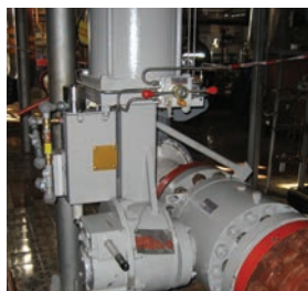
Figure 1 – Control valve installation BEFORE installing ANJ
