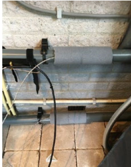
Both PT1000 elements insulated
