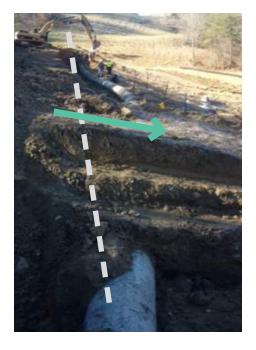
Almost any pipeline can be affected by one or more of the above events but pipelines that are offshore, or in mountainous or geologically unstable areas are at particularly high risk. Pipeline curvature causes bending strain in the pipe wall which can lead to buckles or wrinkles, can exacerbate the significance of other defects especially cracks or even lead to global collapse in severe cases.
