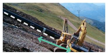
Strain demand is defined as the magnitude of strain acting on the pipeline and will vary along its length depending on the loads acting on the pipeline and the pipe geometry. The strain demand information is a required input into a strain-based integrity assessment of a pipeline section that is subject to a strain from external loads.
