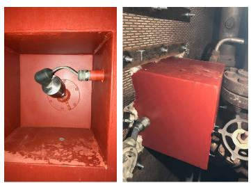
This new cost-effective installation offers the lower cost Flame Tracker option with no water-cooling system needed. Flame Trackers are exceptionally reliable and can be a big improvement over older Geiger Muller-type sensors or other less effective sensing methods. Reuter-Stokes is pleased to share drawings and installation methods with new customers, including the installation of Flame Trackers on turbines with no recessed panels or turbines that include panels.
