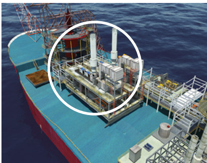
High-Pressure Gas-Injection Compressors
