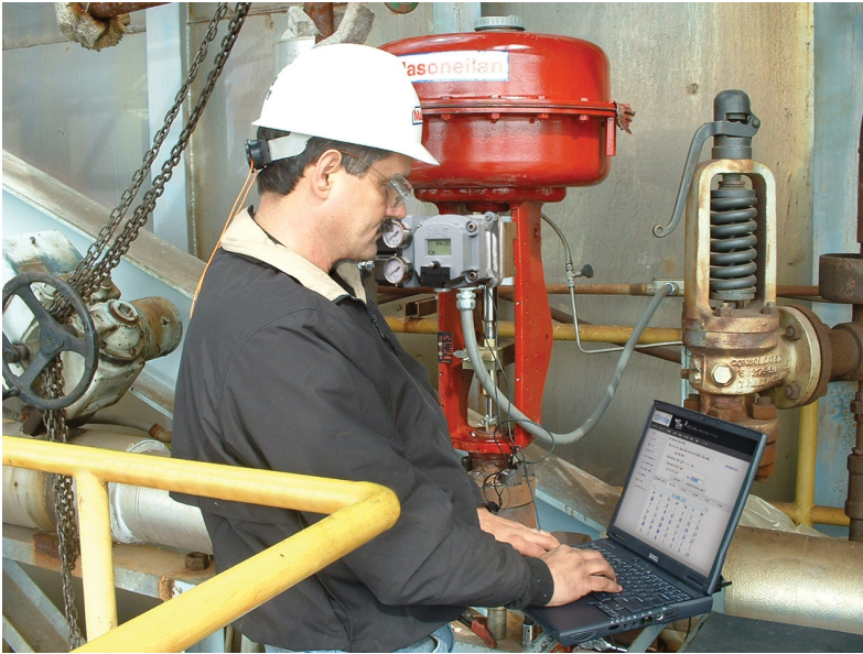
Figure 1. A digital technician setting up valve software to perform an in-situ test on a pressure relief valve.
