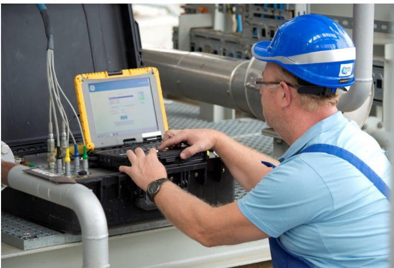
Figure 2. The digital technician is able to test the valve without removing it in addition to seeing its historical performance.
