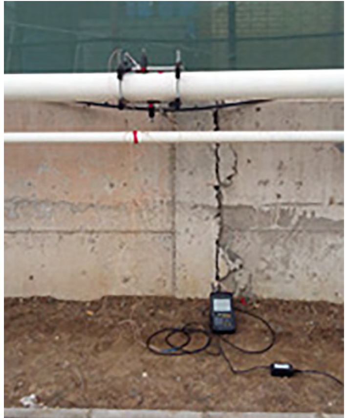
C-RS 401 transducer installation on the penstock
