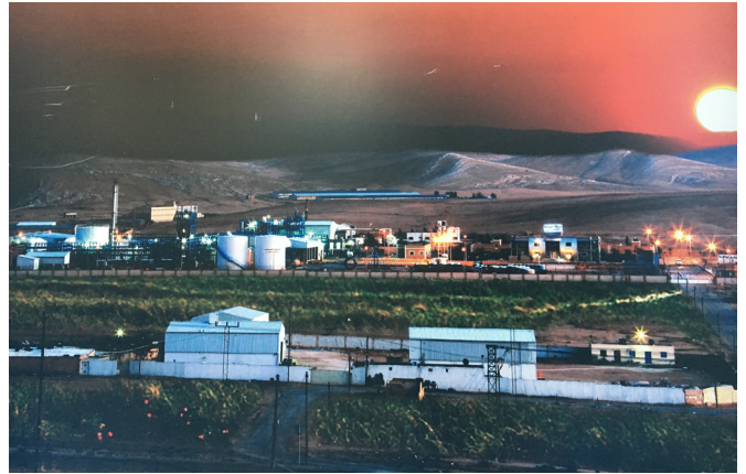
Al-Baha Company for Caustic Chlorine Industries Chemical Plant
