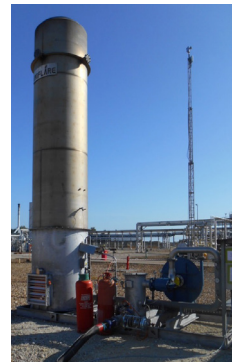
Temporary flare column operating with permanent pilot flame, flame-out emergency shutdown, and LP pressure-regulating valve to allow pigging to continue at higher pressure
