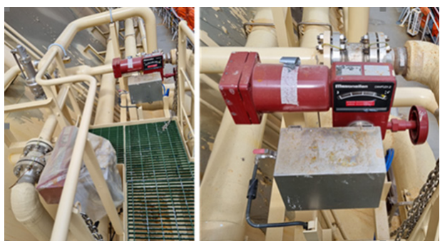
Figure 5. Control valves installed on LNG tankers need to be designed and certified for installation in the harshest of marine environments.
