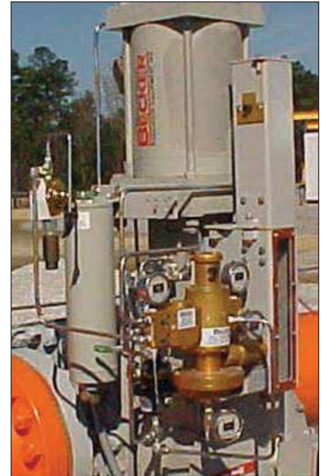
Figure 8 - HPP-4 with VB-250 Volume Boosters The HPP-4 represents a new and improved version of the HPP-2 Positioner. The HPP-4 provides increased sensitivity and process performance with the same Becker reliability. The HPP-4 is typically utilized in high speed applications or scenarios where large volume valve actuators are required. Note that the HPP-4 pictured above incorporates Becker Model VB-250 Volume Boosters. VB-250 Volume Boosters provide additional instrument flow volume capacity necessary for operation of large volume actuators and high speed applications. Additionally, the HPP-4 is shown with Becker’s NBV No-Bleed Valve to completely shut off bleed gas when the control valve is in either the full-open or full-closed position.
