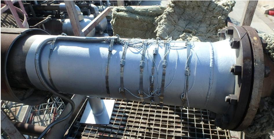
Photo 1 – Installation of UT sensors under insulation (T = 130°C / 266°F)
