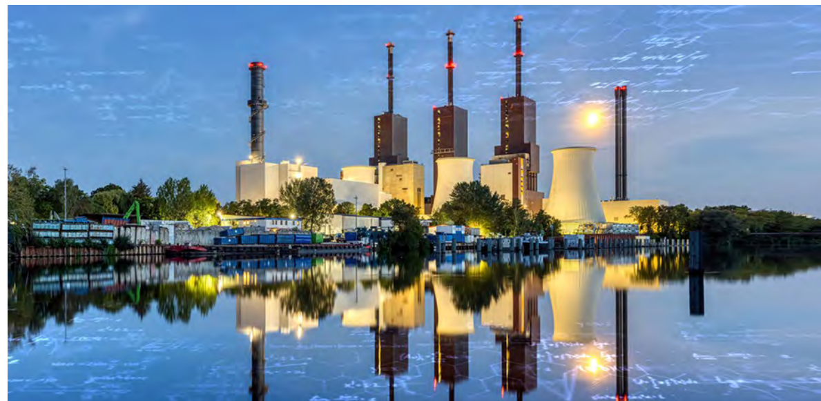
Combined heat and power plant, Berlin, Germany
