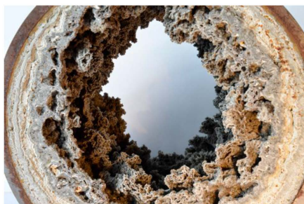
Figure 1—Example of scaling in geothermal wellbore (source: https://geo40.com/geothermal-innovation/ )
