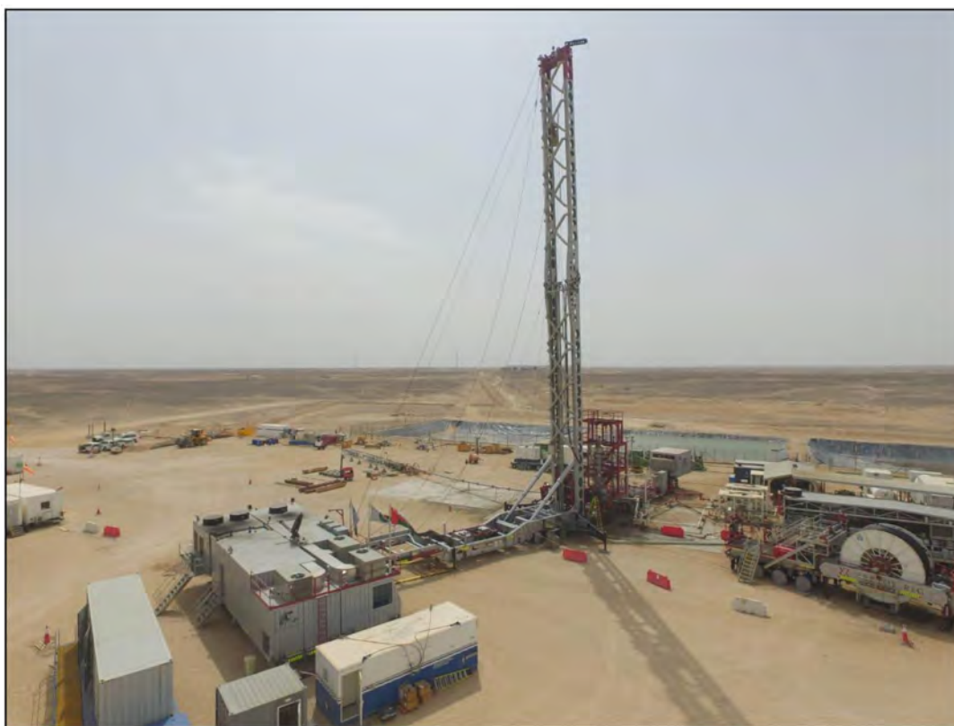
Figure 4—Masted coiled tubing unit designed specifically for UBCTD
