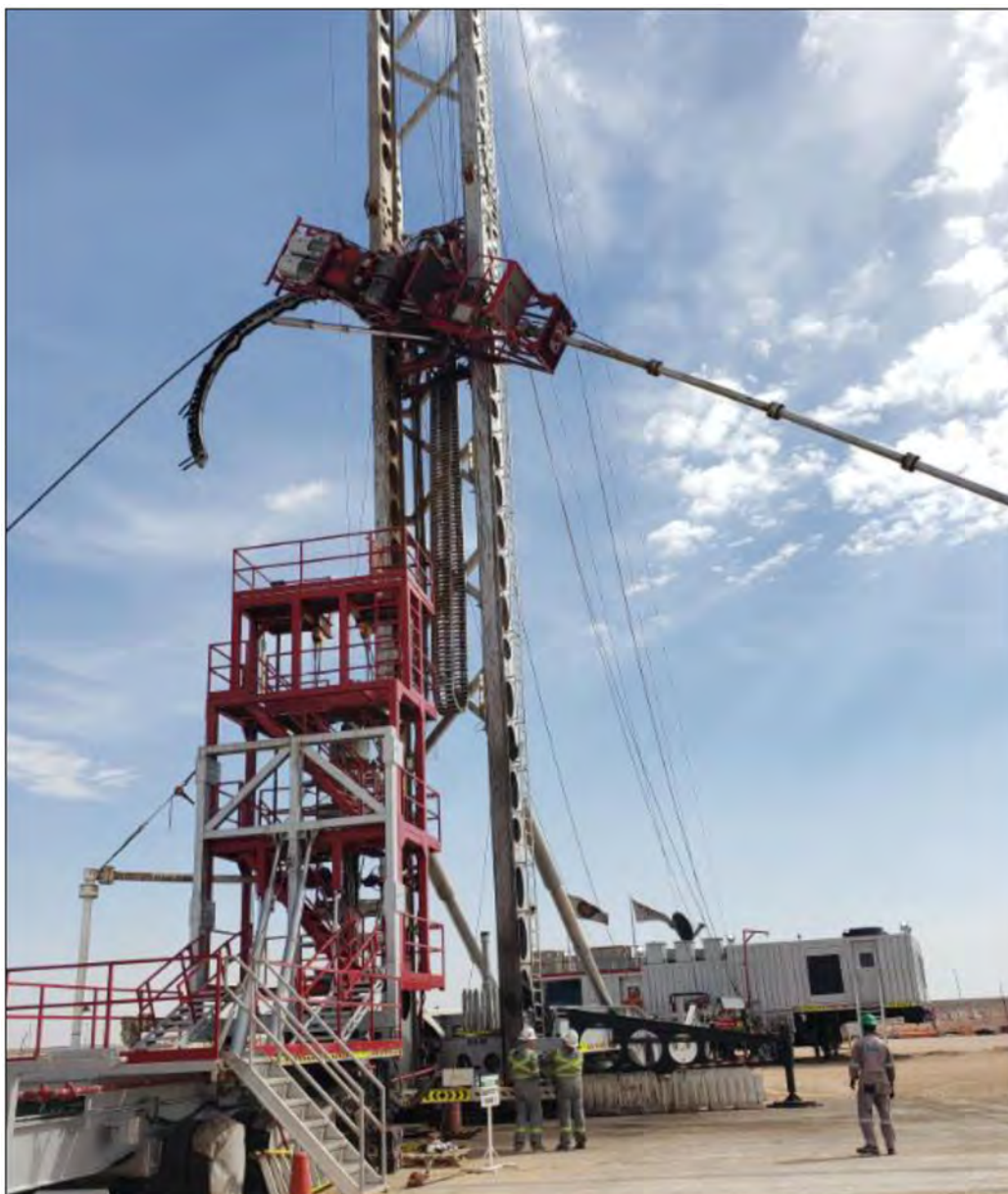
Figure 5—BHA being picked up within lubricator
