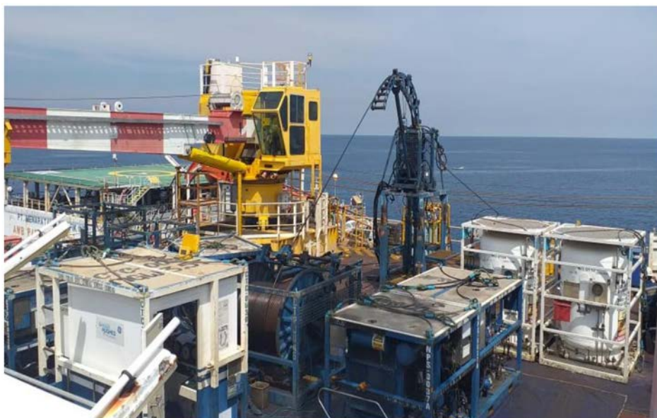
Figure 4—Equipment set up on South Mahakam platform
